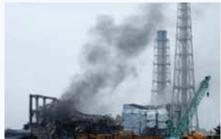
▲ Damage to the Fukushima nuclear power plant after the March 2011 earthquake
