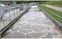
Pulsair Chemical and Wastewater Mixing Systems efficiently mix aeration tanks, anoxic basins, sludge tanks, and chemical tanks using up to 75% Less **Energy** than conventional mechanical mixers...and there are no immersed impellors, shafts, gears, seals or any other moving parts in the tank.
