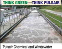
Mixing Systems efficiently mix aeration tanks, anoxic basins, sludge tanks, and chemical tanks using up to 75% Less Energy than conventional mechanical mixers...and there are no immersed impellors, shafts, gears, seals or any other moving parts in the tank.
