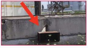
The arrow shows a hole in a containment dike: more damage can be seen at the base and the top of the dike wall. Other examples of damage include cracks in dike walls or floors, holes where pipes have been installed passing through dike walls, and anything else that would allow spilled material to flow out of the dike area.
