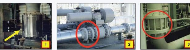
Would you recognize the metal cover (yellow arrow) in Picture 1 as an important piece of safety equipment? If it was damaged or missing, would you know to report it so that it could be repaired or replaced?
