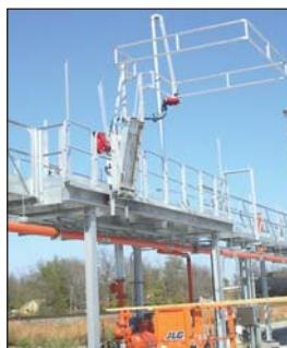
Track mounted gangway can be moved back and forth along the elevated track and extended as necessary to provide safe and easy access or egress from the vehicle no matter what the spotting or configuration.
