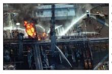
additional stress. This resulted in a brittle fracture of the heat exchanger. A vapor cloud estimated to contain more than 10 tons of flammable gas was released, and subsequently ignited by a heater. The explosion and fires killed 2 workers, injured 8 others, and the fire burned for 2 days. The gas supply to a large part of Australia was disrupted for nearly 3 weeks, impacting the lives of an estimated 4 million people. Total economic loss was estimated at over \$1 billion Australian dollars.
