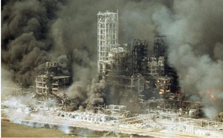
Figure 1: The fires after the explosions took 10 hours to be brought under control (ref 1)
