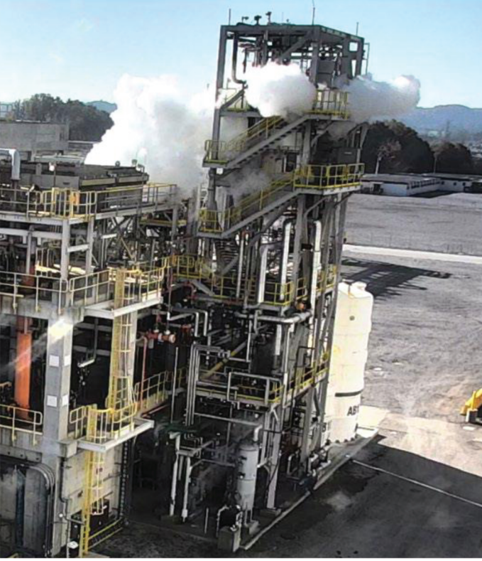
Figure 1. The platform where the release occurred. Fifteen seconds later, the structure was engulfed by the cloud. (Ref CSB report No. 2021-01-I-TN)
