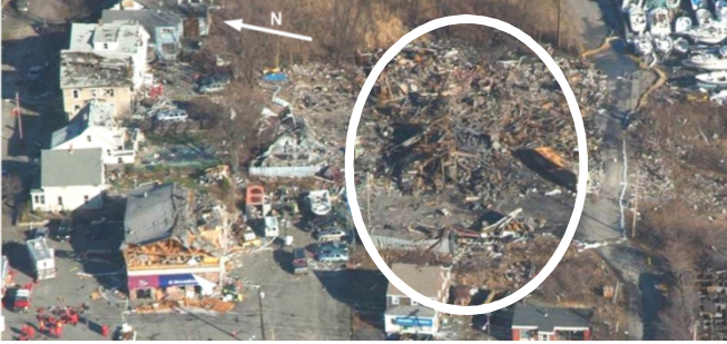
Figure 1 Paint plant Explosion damage
