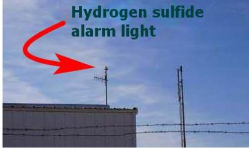
Fig. 2: H<sub>2</sub>S alarm warning light
