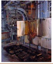
The investigation revealed that the some of the materials in the containers were incompatible and, over time, chemicals had leaked from damaged containers, overfilled containers, or from spills on the outside of containers. Some of this material fell through the open grate floor into a cable tray below the floor. It was difficult to see the spilled material in the cable tray, or to clean it up, and eventually some of the spilled materials reacted, got hot, and burst into flame.
