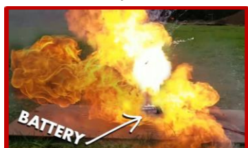
Figure 2: Lithium-ion battery fired demonstration.
