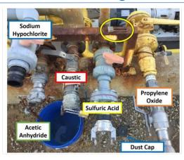
Figure 1: Connections to chemical tanks at MGPI. Sulfuric Acid fill line padlock (circled) on the metal frame. Sodium hypochlorite dust cap on the ground. (ref CSB report 2017-01-I-KS)
