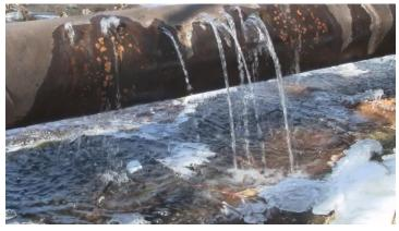
A company decided to stop making a chemical product. One of the input materials was toxic and corrosive phosphorus trichloride (PCl<sub>3</sub>). The lines to the storage tank and the process area were cleared of PCl<sub>3</sub>. A few years later, an operator found a leak outdoors. The investigation found that the leak was coming from the "empty" PCl<sub>3</sub> line. No one was injured and the spill was contained.
