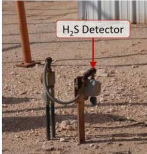
Fig. 1: One of the H<sub>2</sub>S detectors
