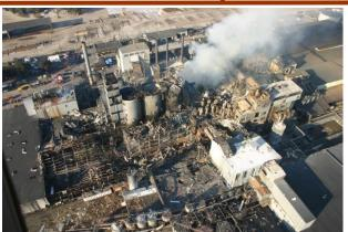
Sugar is combustible; while it is hard to ignite, explosions provide more than enough energy to cause damaging explosions and fires.
