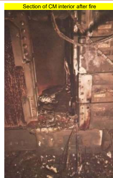
Section of CM interior after fire
