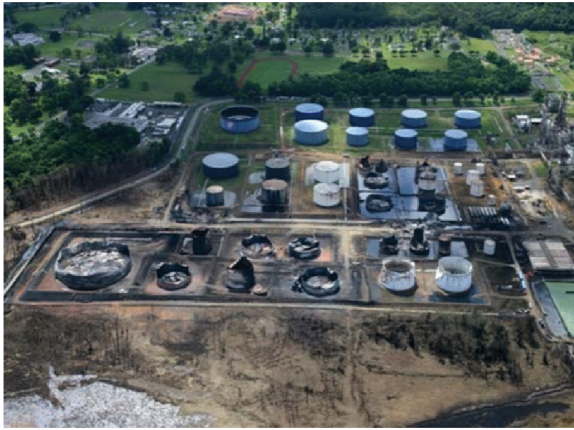
Damage to the facility after the fire
