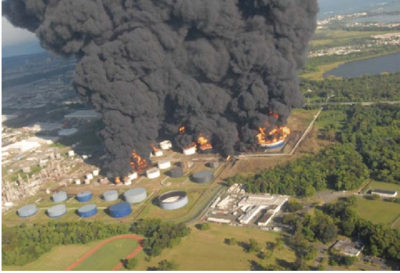
Multiple tanks burning in the fire
