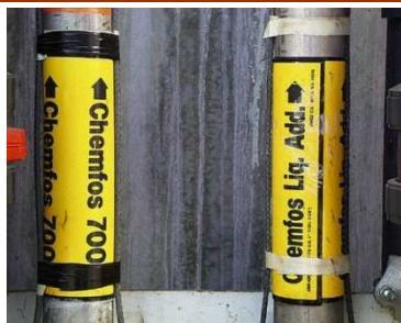
Similar labels on these pipes contributed to unloading the wrong material into a storage tank. A chemical reaction resulted, releasing a toxic gas which injured 6 people. See the April 2012 Beacon.
