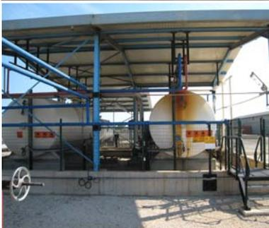
Most people recognize that containment dikes around storage tanks, and sloped containment pads for pumps, process buildings and structures, truck and rail car unloading areas, and other potential spill locations have an important environmental protection function – preventing contamination of soil and surface water. But, do you know that they often also have important safety functions? Some examples include:
