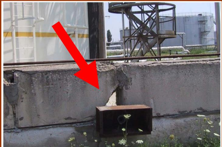
The arrow shows a hole in a containment dike. More damage can be seen at the base and the top of the dike wall. Other examples of damage include cracks in dike walls or floors, holes where pipes have been installed passing through dike walls, and anything else which would allow spilled material to flow out of the dike area.
