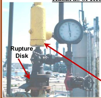
A vessel has a rupture disk and a pressure relief valve in series to protect against high pressure in the vessel. There is a pressure gage on the pipe between the rupture disk and the relief valve. As a part of your regular plant inspection, you are supposed to check the pressure gage. The gage normally reads zero. Today you observe a pressure of nearly 50 psig (~3.5 barg) as shown.
