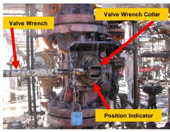
Many people would expect this valve to be closed - the position of the valve handle (in this case, a "valve wrench") is perpendicular to the pipe. But close inspection of the valve position indicator shows it is parallel to the pipe, clearly indicating the valve is open! WHY? The valve wrench collar is square and can be positioned in two ways – one with the valve wrench parallel to the valve position indicator and the other with the valve wrench perpendicular to the position indicator.
