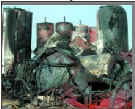
Acidente investigado e foto fornecida pelo U.S. Chemical Safety and Hazard Investigation Board. Visite o site t http://www.csb.gov
