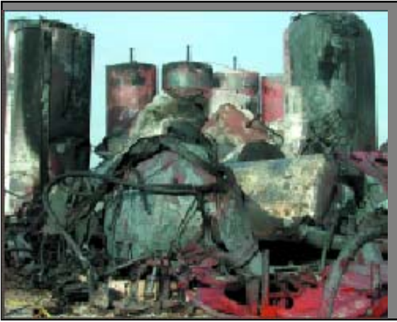
This accident investigated by and picture provided by the U.S. Chemical Safety and Hazard Investigation Board. Visit their site at http://www.csb.gov
