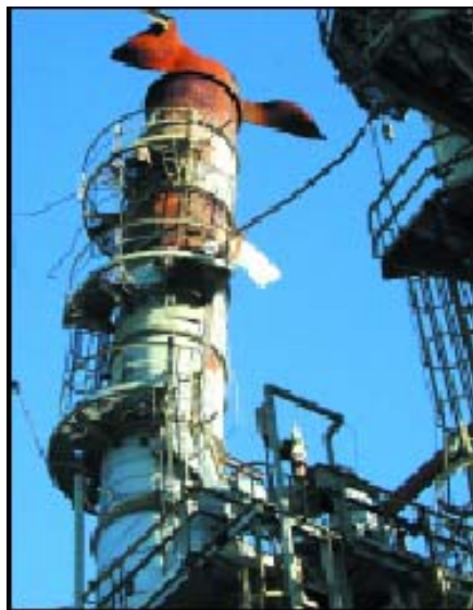
This accident investigated by and picture provided by the U.S. Chemical Safety and Hazard Investigation Board. Visit their site at http://www.csb.gov
