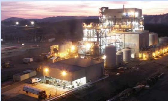
Last month, DuPont officially christened its $100-million facility in Loudon, TN, which is using a proprietary fermentation process to produce 1,3-propanediol from corn sugar instead of petroleum-based feedstocks. Source: DuPont.
