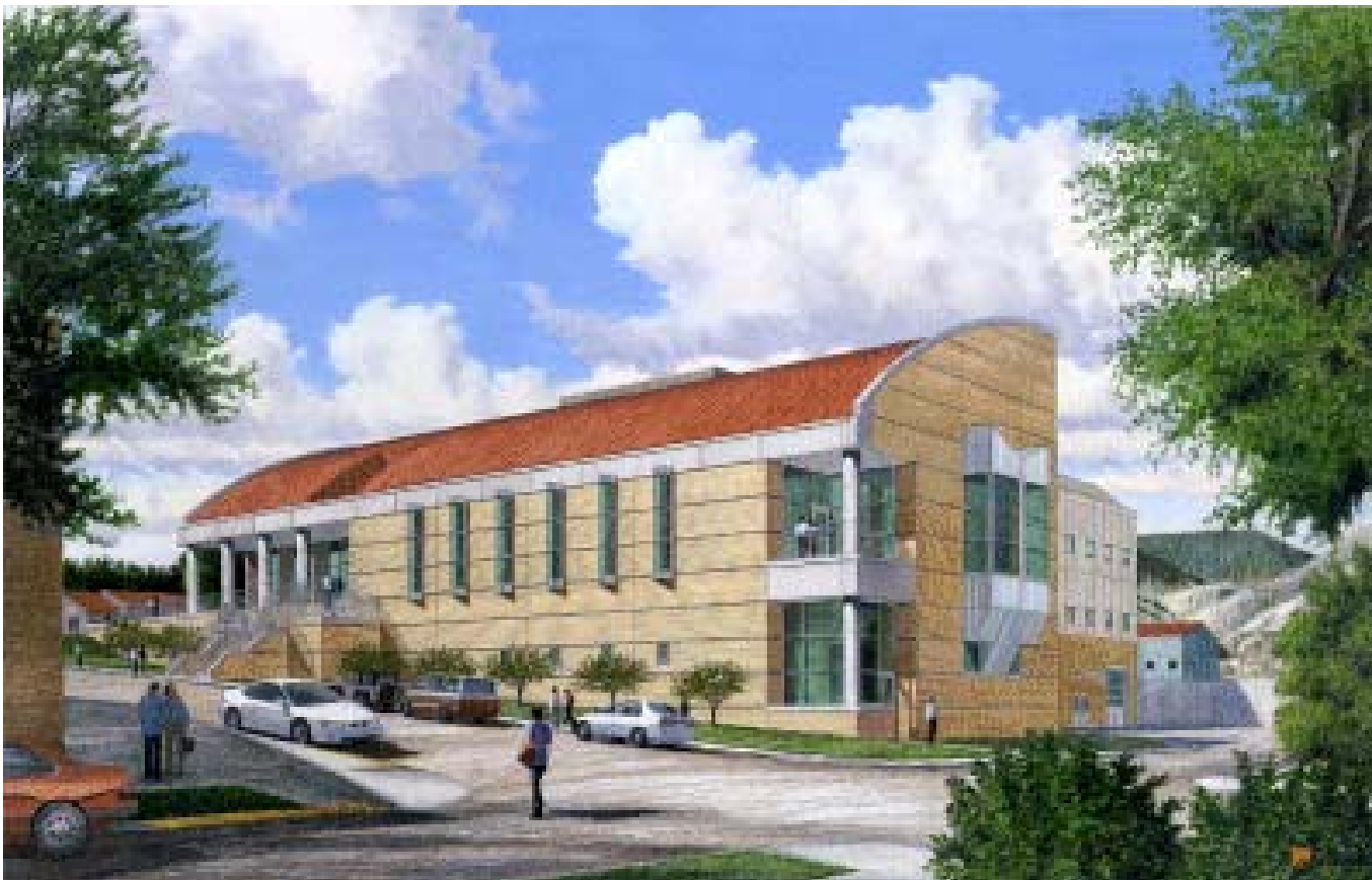
Photo of the east face of the Colorado School of Mines Geology Museum
