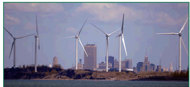
The former Bethlehem Steel plant in Lackawanna, NY, is now home to the Steel Winds wind farm.
