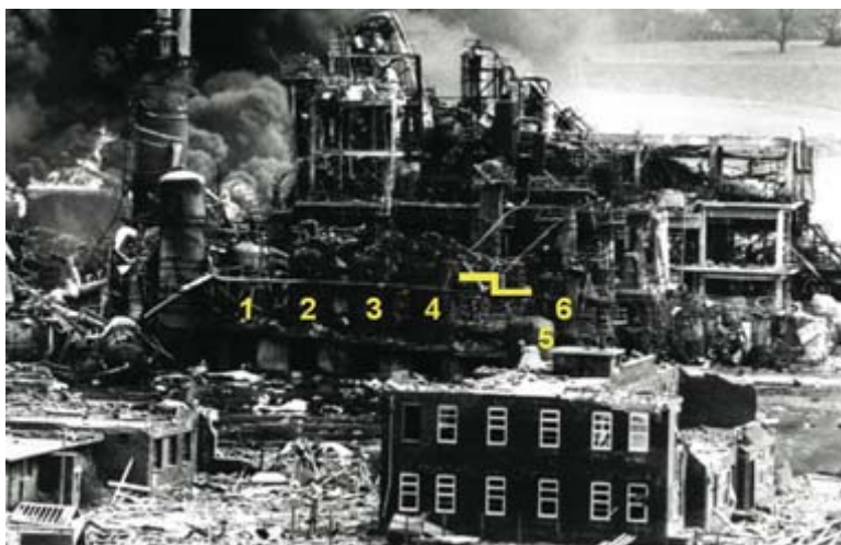
Figure 1: Dutch State Mines Nypro Plant in Flixborough, UK after the deadly 1974 explosion.
