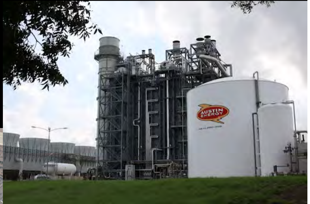
Sand Hill Energy Center, Austin, TX Credit: Austin Energy
