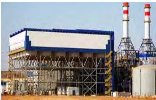
Dry-Cooled Power Plant
