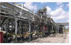
mixture, at an estimated pressure of 70 psig, contained flammable vinyl chloride. The operator was not able to open the pneumatic valve on the bottom of the reactor — there was a safety interlock that prevented the valve from being opened while the reactor was under pressure. It is also believed that the operator connected a nearby air supply to the valve and forced it to open, releasing the reaction mixture into the building. Flammable vapors from the released material ignited.
