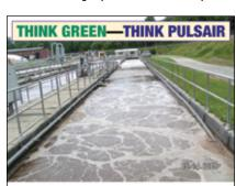
Pulsair Chemical and Wastewater Mixing Systems efficiently mix aeration tanks, anoxic basins, sludge tanks, and chemical tanks using up to 75% Less Energy than conventional mechanical mixers...and there are no immersed impellors, shafts, gears, seals or any other moving parts in the tank.
