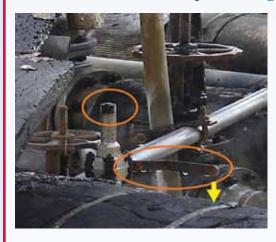
piece of debris fell from temporary scaffolding used to support people and material. It hit the straight handle of a quarter-turn ball valve that served a <sup>3</sup>/<sub>4</sub>-in. (about 20 mm) vent on a large process pipe. The falling debris caused the vent valve to open. The pipe contained flammable material, which was released through the vent. The released material ignited, and the resulting fire killed one contract worker and seriously burned two others.
