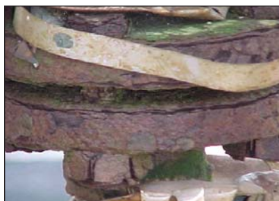
April — Mechanical integrity
