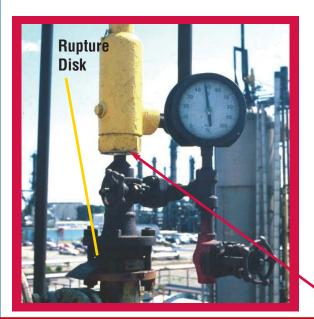
A vessel is equipped with a rupture disk and a pressure relief valve in series to protect against high pressure in the vessel. There is a pressure gage on the pipe between the rupture disk and the relief valve. As a part of your regular plant inspection, you are supposed to check the pressure gage, which normally reads zero. Today you observe a pressure of nearly 50 psig (~3.5 barg), as shown in the photo.
